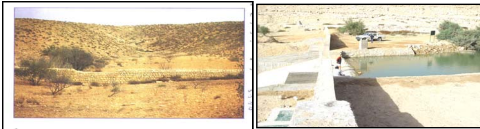
Figures (4) Stored and productively used runoff of catchment system in the RWH.
