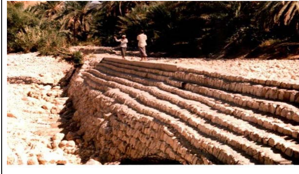
Farmer improved spate irrigation structures in the Hadramawt in Yemen Diversion Weir with a stepped downstream face
