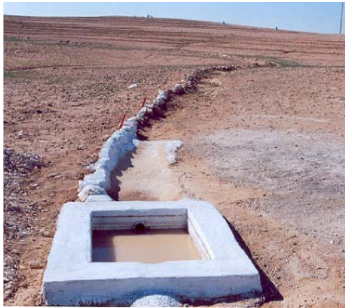
Maintaining collecting wells
