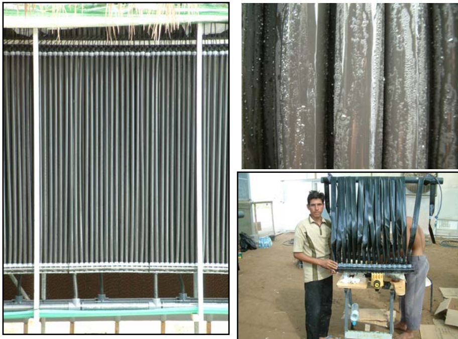
Assembly on site of the 'Watermaker' all plastic condenser.
