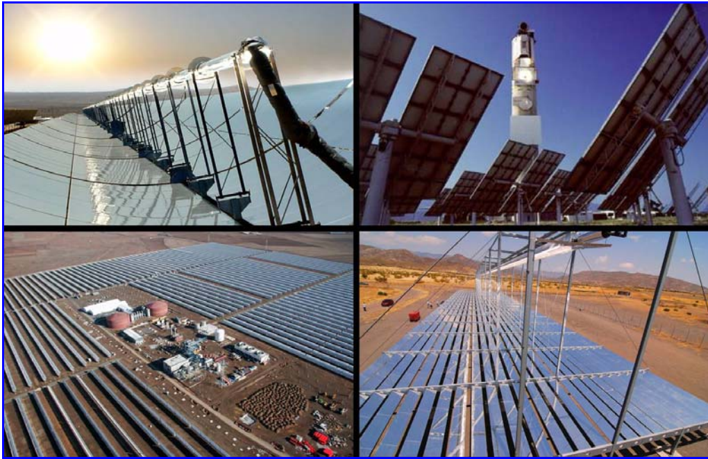
Figure 1: Mainstream concentrating solar power solar field technologies for the production of high-temperature solar heat for power generation and seawater desalination via thermodynamic cycles and process steam: parabolic trough concentrating solar thermal collector (top left), heliostat field in front of a solar central receiver tower (upper right), parabolic trough field around a steam cycle plant with night-time energy storage (bottom left), linear Fresnel collector (bottom right). Sources: Schott AG, PSA, ACS Cobra, MAN/SPG
