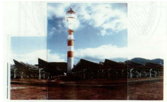
Fig. 5 Solar power plant of beam-down type
