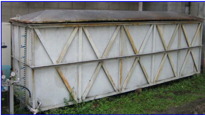
Figure 1: General view for the tank
