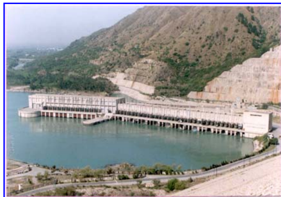
Figure 4: Tarbela Power House
