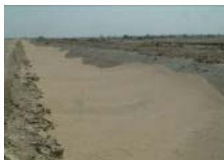
Buried water canal by sand
