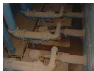
Sand entrance to infrastructures
