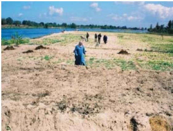
Photo 4: Low land heightened by dredged material in Damietta branch
