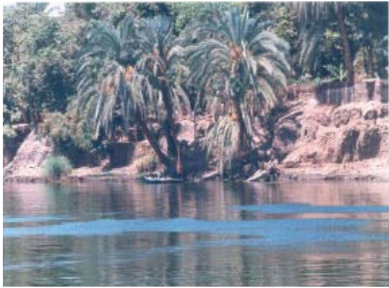
Photo 3: Steady progressive soil erosion reveals the root of palms
