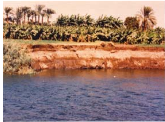
Photo 2: land erosion due to seepage effect
