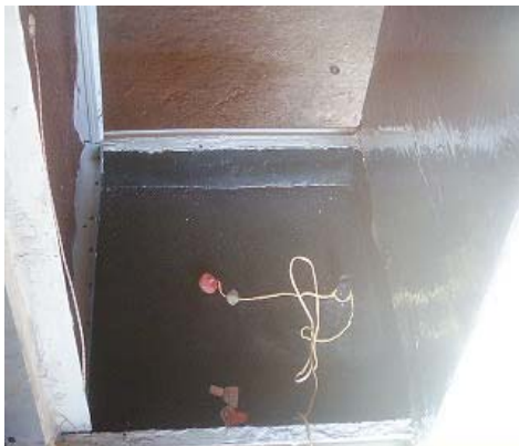
Fig. 3: lower basin under construction
