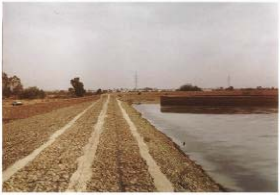
Fig. 1: Storage / Recharge Reservoir
