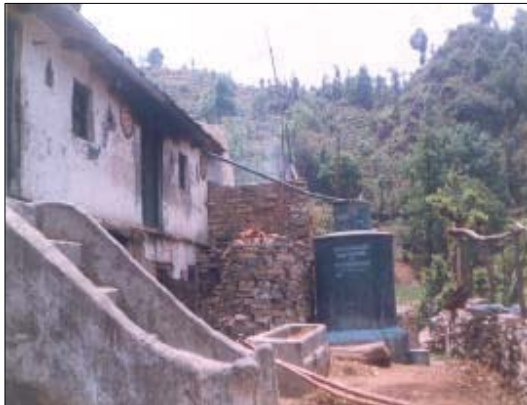
Fig. 1: Rooftop rainwater harvesting
