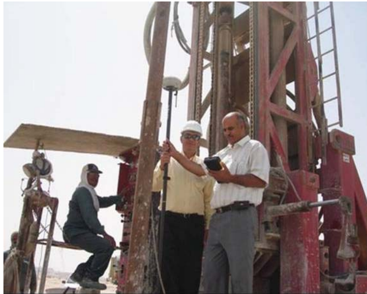
Fig. 18: Following up of Wells drilling program by the authors based on the 2-D resistivity results
