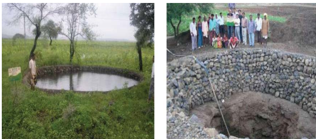
Fig. 8: Dug wells recharged by in situ water harvesting
