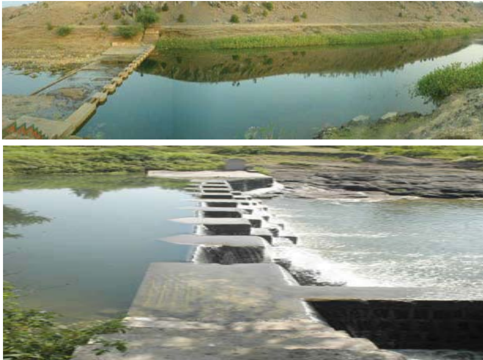
Fig. 6: Check Dams in Rajasthan, India
