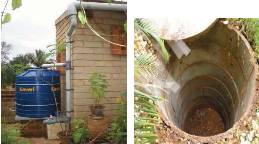
Fig. 5: a) The Rain Barrel - a simple method of rainwater harvesting b) A recharge well
