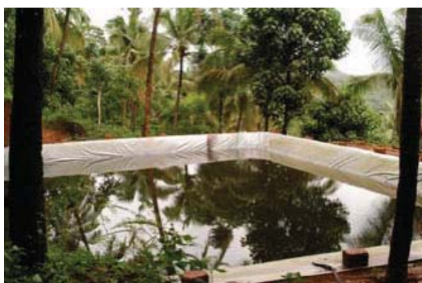
Fig. 9: UV-resistant, plastic-lined rainwater harvesting tank for irrigation.
