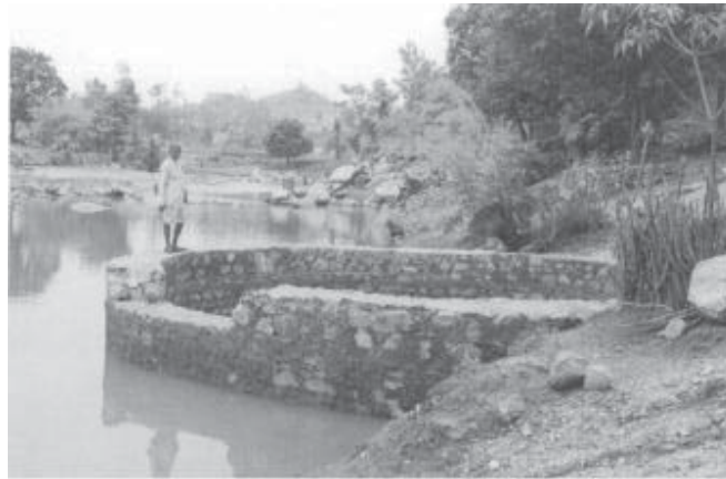
Fig. 4: Recharging through Naal bandhana - subsurface well recharging structure
