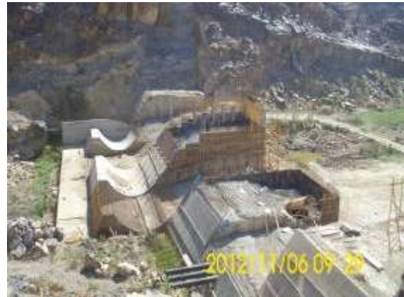
Fig. 6: Terjis Dam Project
