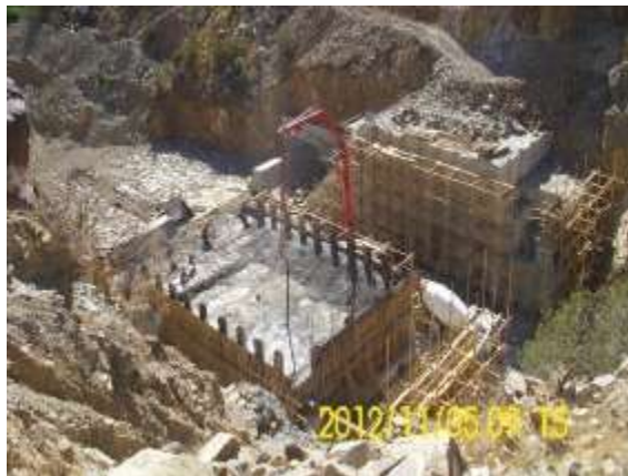
Fig. 5: Halba Dam Project
