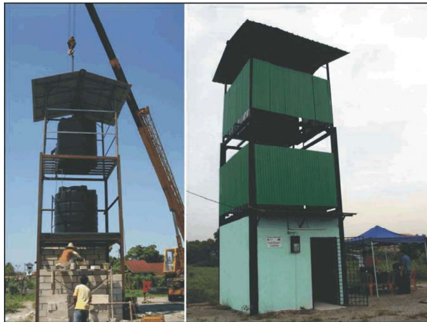
Fig. 2: Construction of the in-situ treatment plant.
