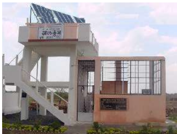
Plate 1: Electrolytic Defluoridation Plant at Dongargaon.
