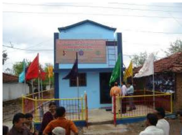
Plate 2: Electrolytic Defluoridation Plant at Sargapur.
