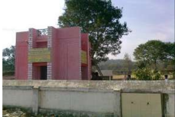
Plate 4: Electrolytic Defluoridation Plant at Malgaon.
