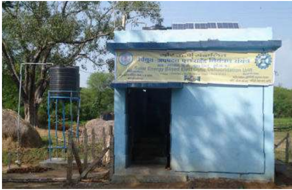
Plate 3: Electrolytic Defluoridation Plant at Usarvara.
