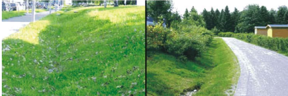
Fig. 3: Trench furrow infiltration in Germany [15]
