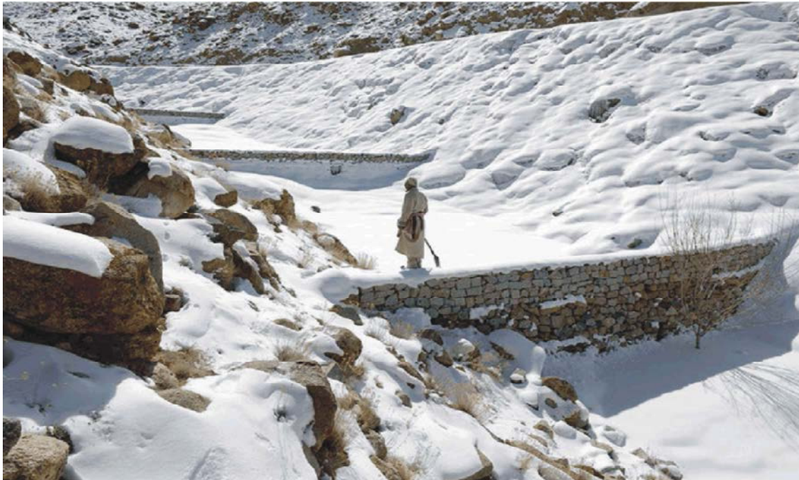
Pic. 1: Artificial glacier at 3,900 m (about 12,800 ft), located above the village of Nang, Ladakh. The cascade is composed of a series of loose masonry walls ranging in height from 2 to 3m, which help freeze water for storage
