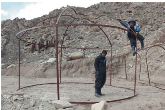
Dome shaped iron bar structure
